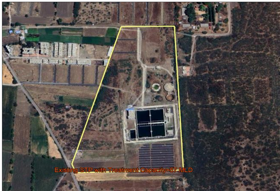
Figure 7-4 Existing Sewage Treatment Plant
